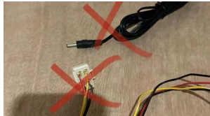
Figure A-7: No connection of wires
